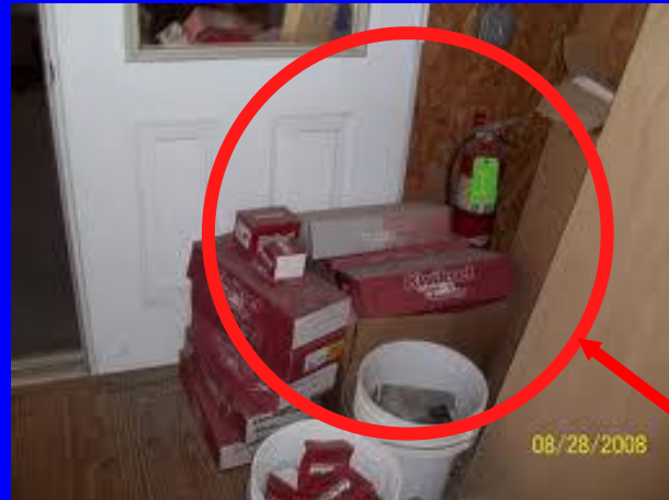
Blocked extinguisher
