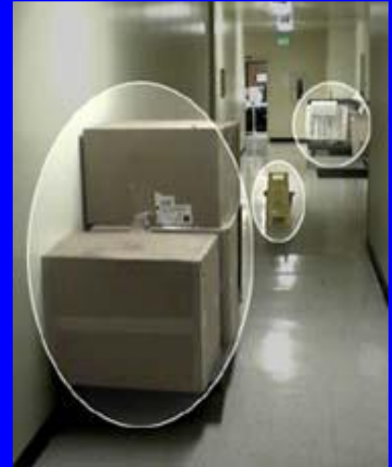
Obstructed exit route
